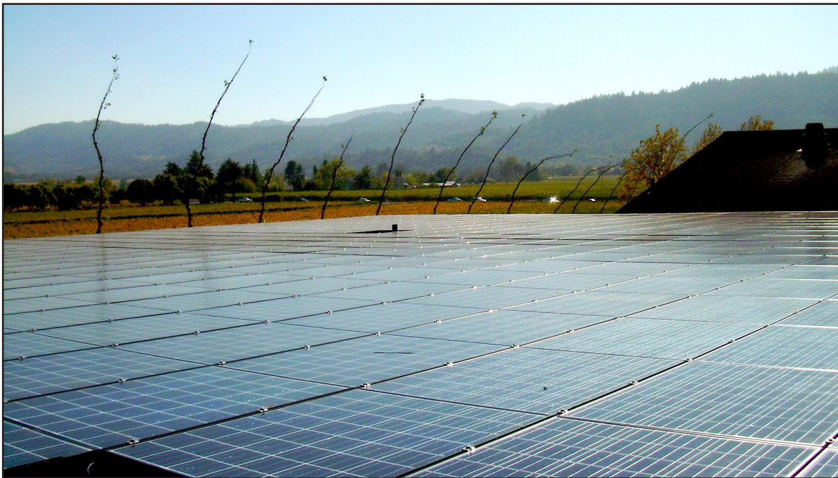
The view of the new solar panel rooftop at Peju.
